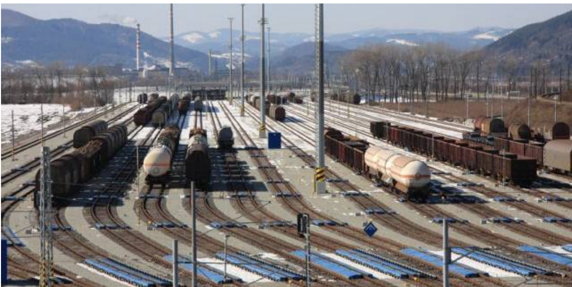
Figure 31: Marshaling yard at Žilina-Teplička, Photo: ŽSR
